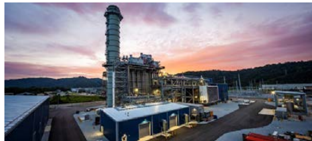
Long Ridge Energy Terminal and GE Gas Power have announced a successful first step to transition the HA-powered facility to carbon-free hydrogen with multiple successful hydrogen demonstration tests in 2022.
