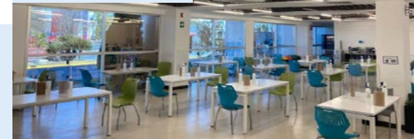
LED lighting installation in Monterrey, Mexico
