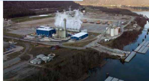
Long Ridge Energy Terminal and GE commissioned and demonstrated the first advanced class hydrogen-burning power plant worldwide using GE's HA Gas Turbine.
